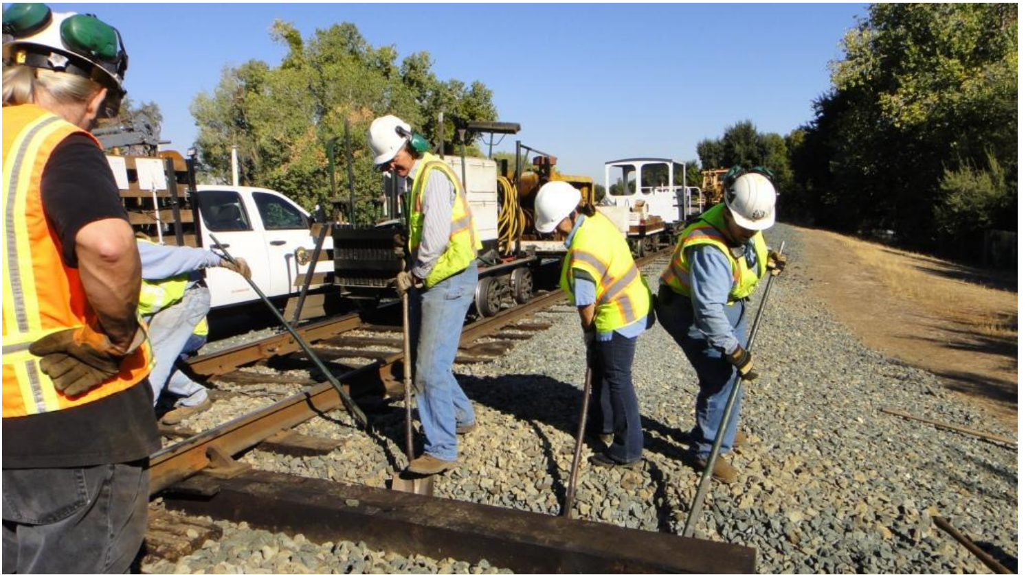
Precision placement: Steve, Pam, and Heather shimmy the new head-block around to make sure it is in the precise spot
