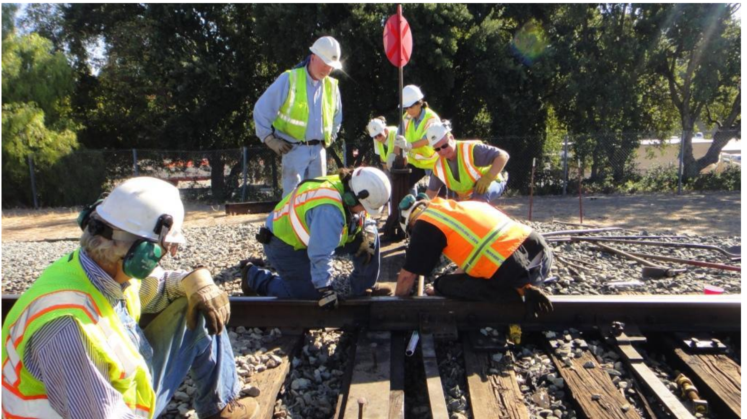
Steve sets spikes in the gauge-plate while Heather and Fred attach the control-rod to the connecting-rod. Ed positions the other end of the control-rod onto the switch stand which Pam holds steady while Clem nips the end of the head-block.
