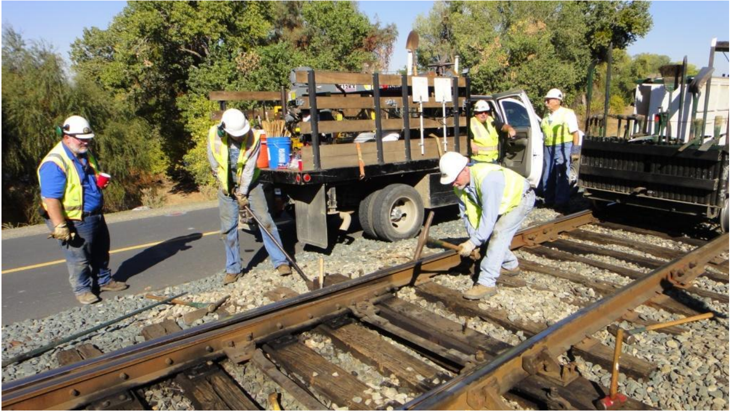
Mike M. spikes the gauge-plate down while Steve nips the head-block
