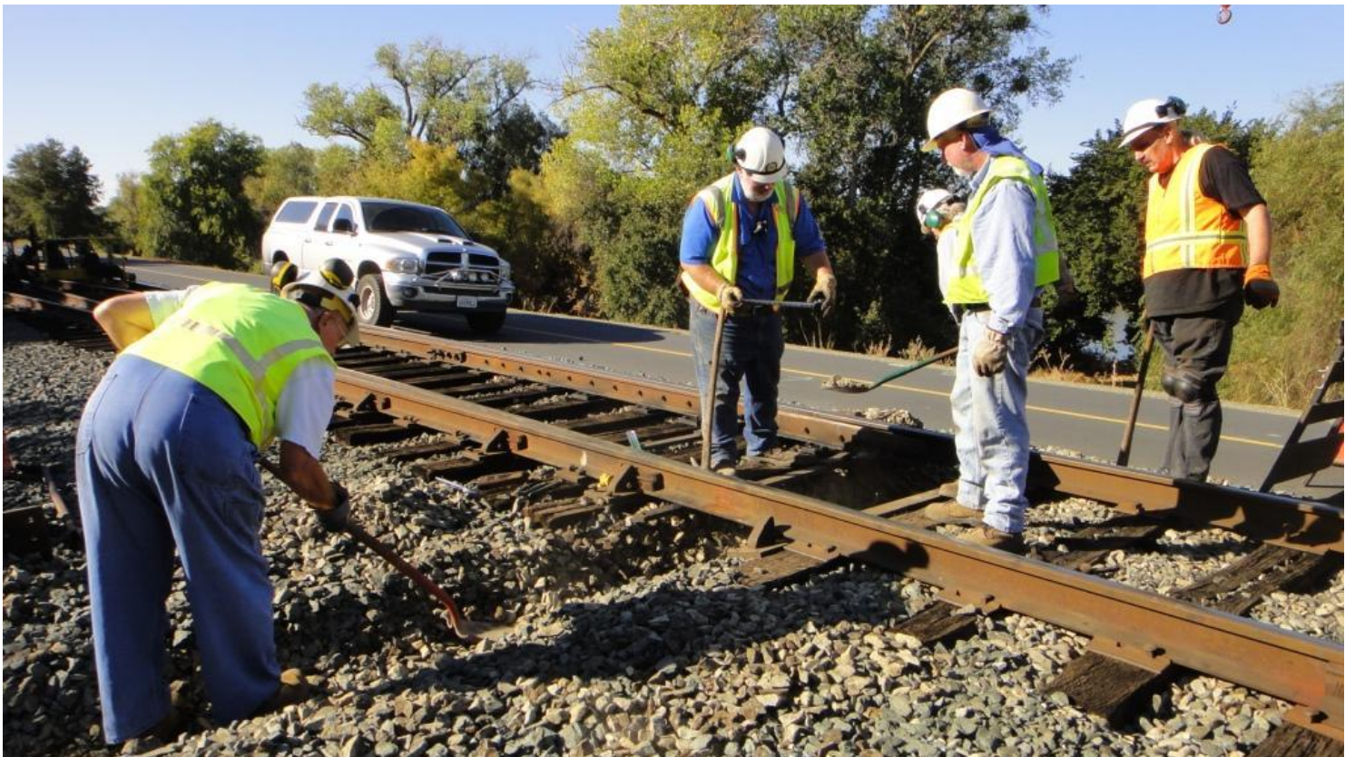
The old cracked head-block is removed and Clem, Frank, Mike, Steve, and Fred dig out the crib to make room for the new head-block
