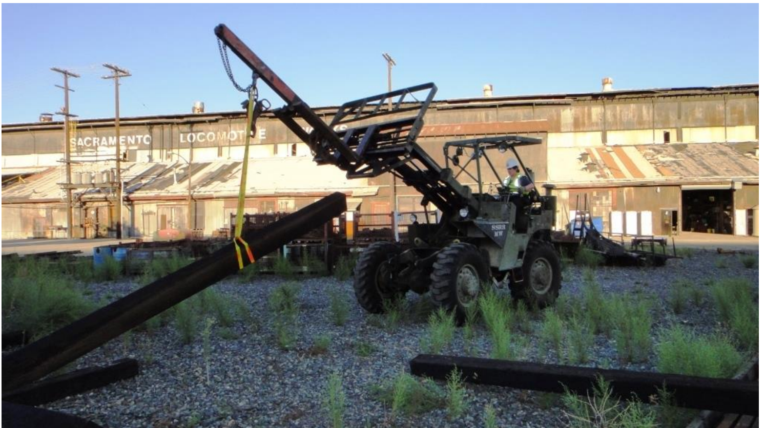
Heather finds a head-block to replace the cracked one down at Switch 17, the north switch at Baths
