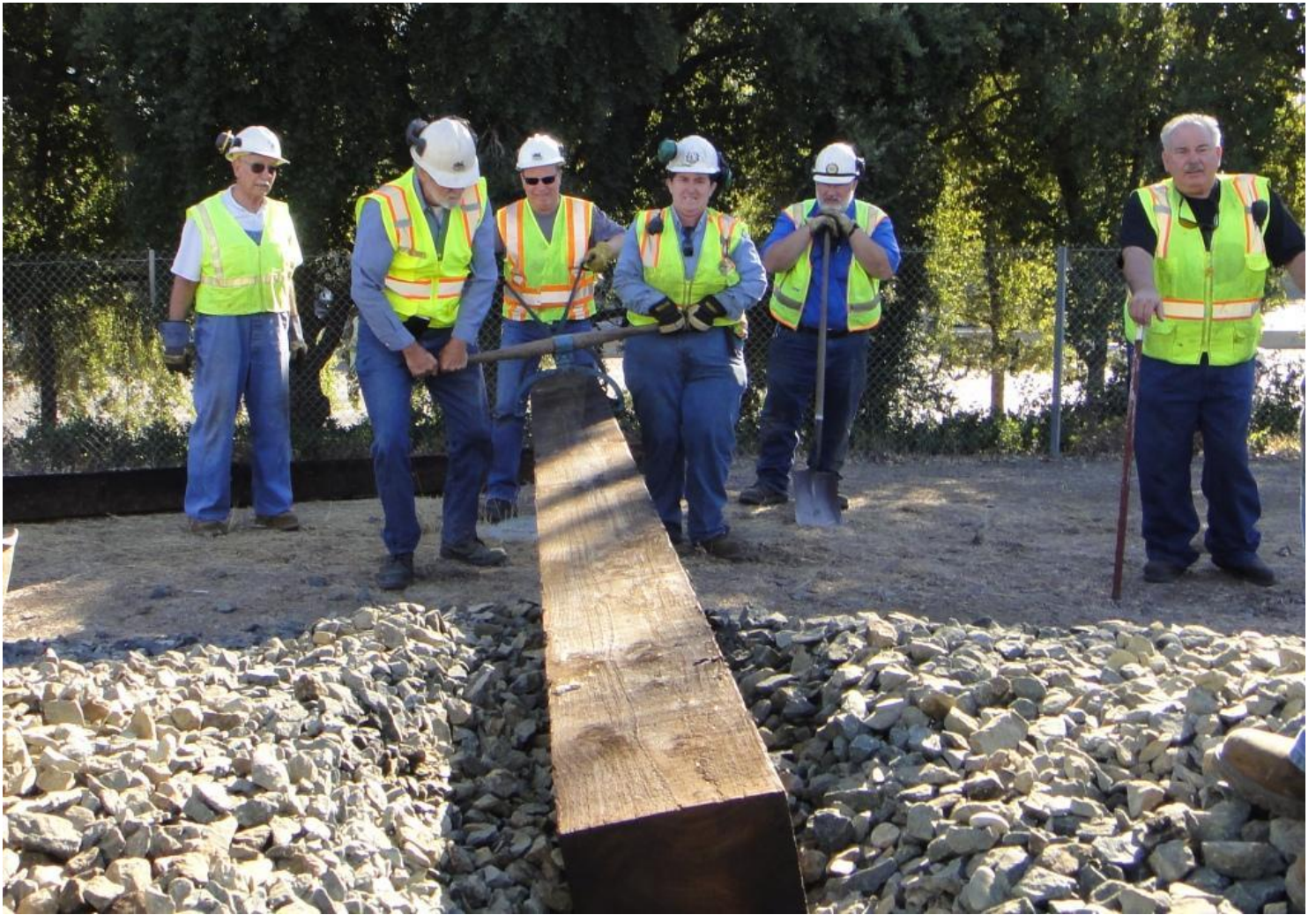
Using timber-tongs and tie-tongs, Alan, Ed, and Heather position the head-block for insertion
